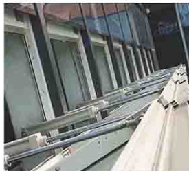
Bottom Hung Windows Installation
